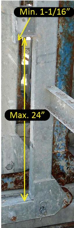
Check the lip of the Walk Thru C-stirrup that hooks onto the midrail. It should be sticking out 1-1/16" with a 1/16" tolerance. If too short it will not properly lock onto the midrail and the stirrup can slip off.
