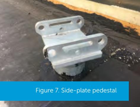
Figure 7. Side-plate pedestal
