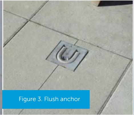
Figure 3. Flush anchor
