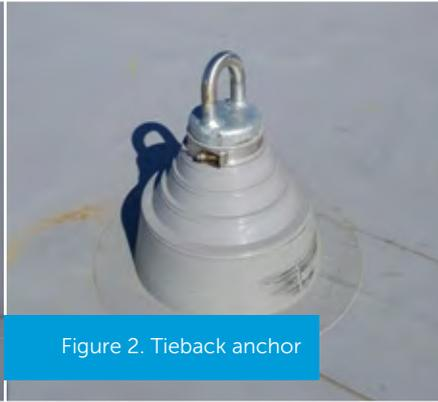
Figure 2. Tieback anchor
